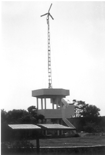
Figure 1. Installed Virya 3.3 turbine (height=20m)
